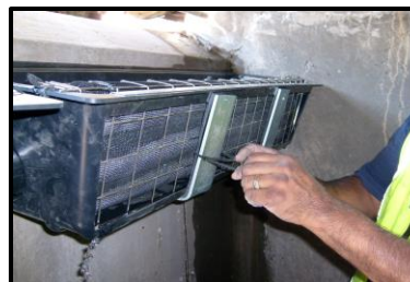
(Filter Cradle Brackets being installed)
