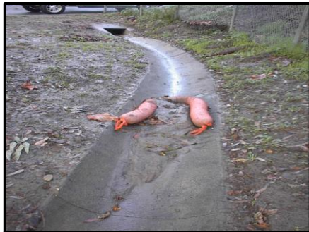
Erosion control for Trench or V-ditches
