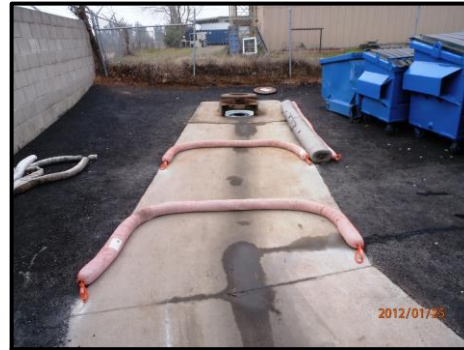
Multiple filtered stages First Wattle: Heavy/large pollutants Second Wattle: Finer filter polishing
