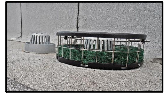
REM Model RDF-14 (4.5") installed on a domed roof drain
