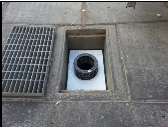
TRITON BFTG Drop Inlet Installation
