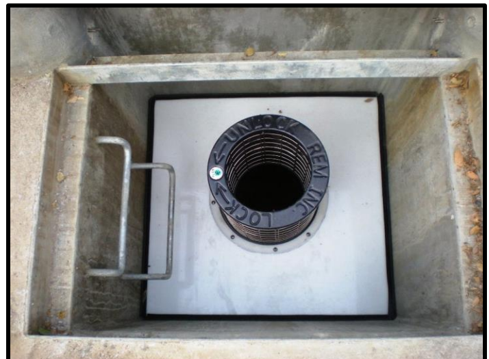
TRITON BFTG Installed with Ladder Rungs
