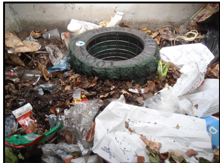
TRITON BFTG field photo (FTC device requires maintenance)
