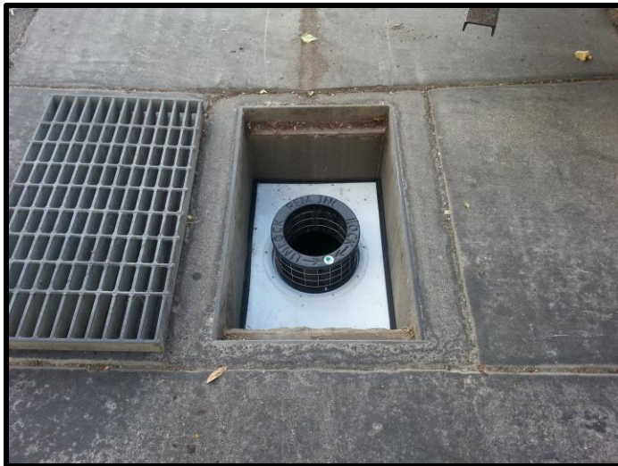
TRITON BFTG Drop Inlet Installation
