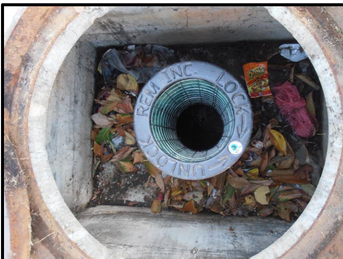
TRITON BFTG Curb Inlet Installation field photo
