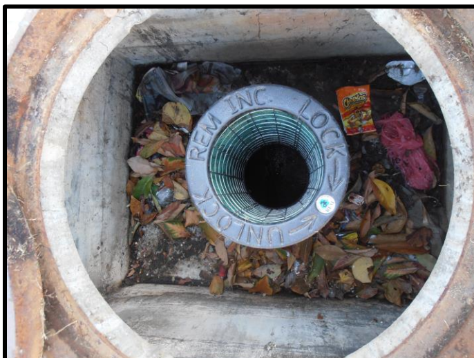
TRITON BFTG Curb Inlet Installation field photo
