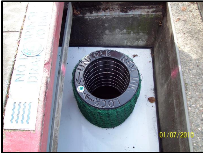
TRITON BFTG - Combo Grate & Curb Inlet Installation
