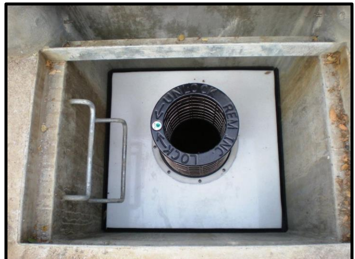
TRITON BFTG Installed with Ladder Rungs
