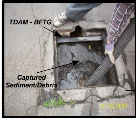
TDAM - Installed, before service
