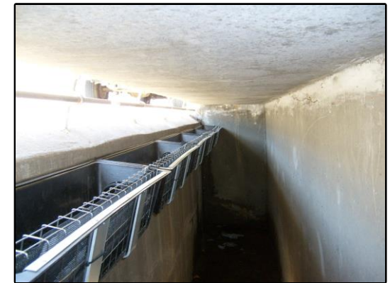
TRC14 - FOG (14' Curb Inlet Filter – Installed)
