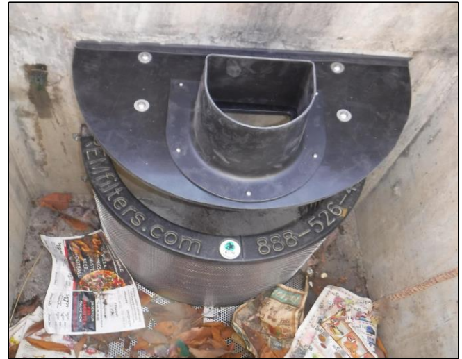
Standard REM CPS-PERF FTC device installation
