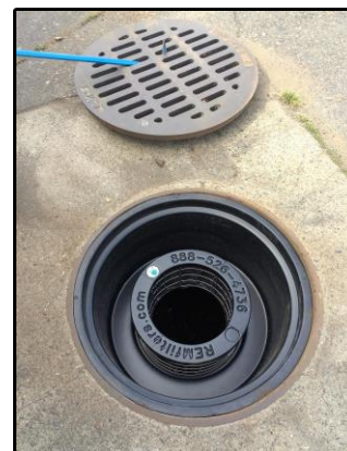
TR24RD-PERF Installed
