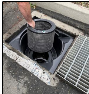
TR2424 Removing Screen
