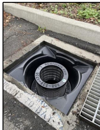
TR2424-PERF Installed
